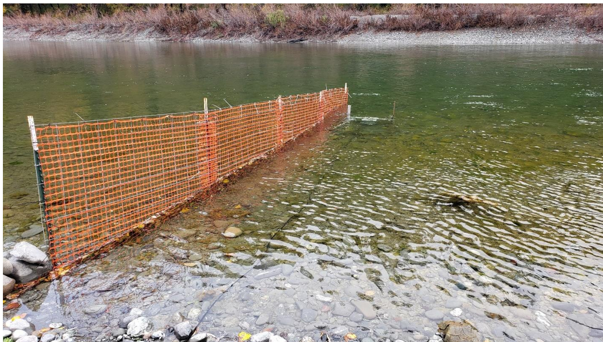
5.) 12.01.2019. Panels with buildup that must be removed early during season. As flows increase, detritus gets flushed downstream and eventually stops collecting on panels.
