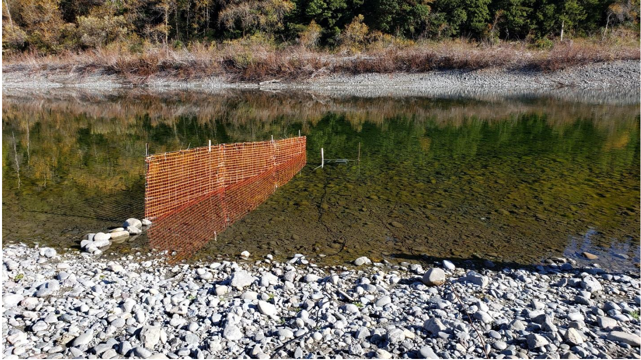
1.) 11.21.2019. Camera in position with installed picket weir and rock wall.
