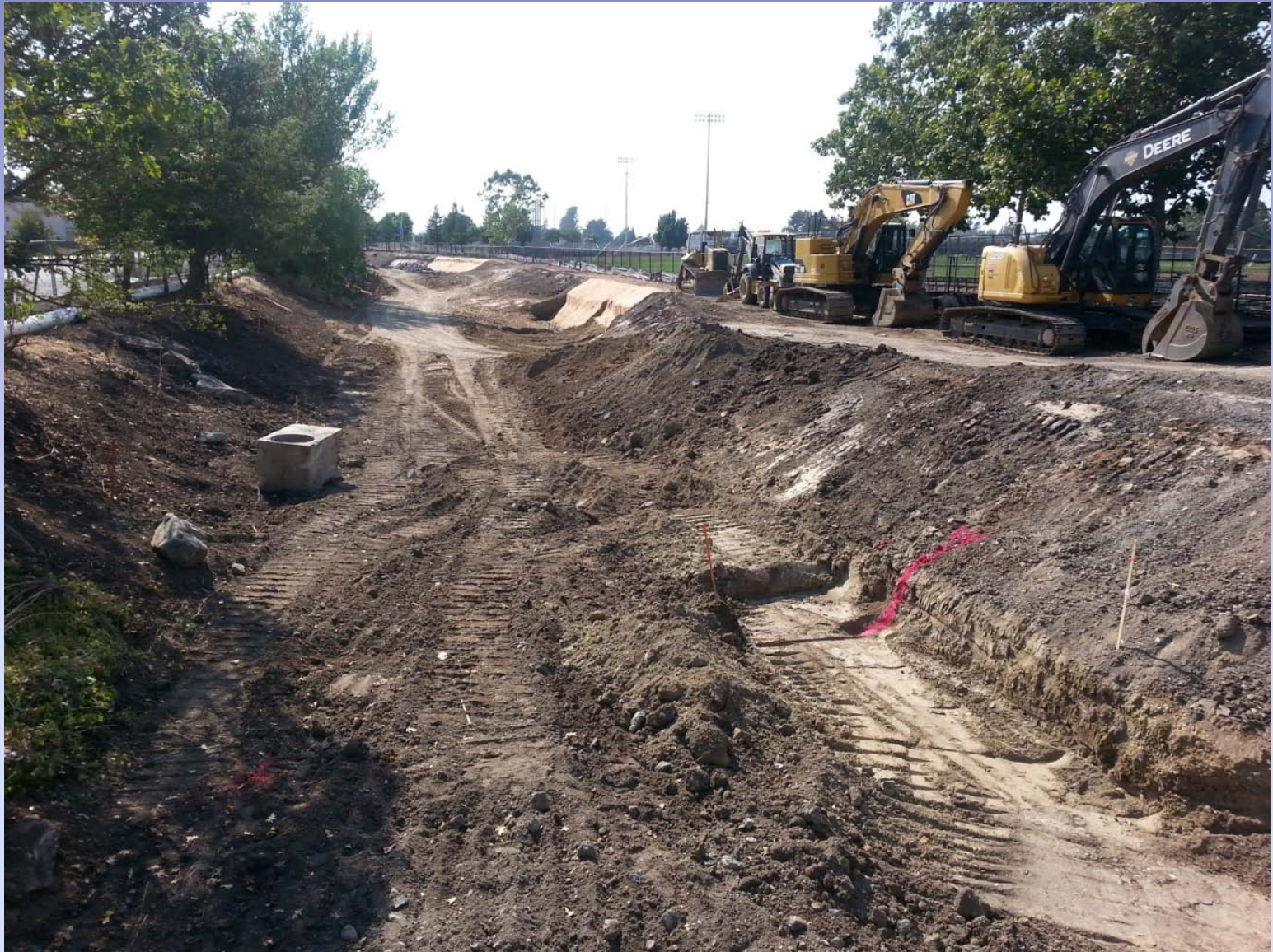
Widening the channel and sloping the bank.
