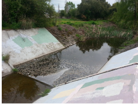
Victoria Drive site, with concrete aprons
