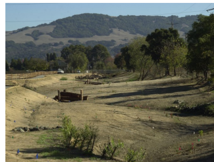
View upstream towards Dutton Meadow after stream widening and re-contouring
