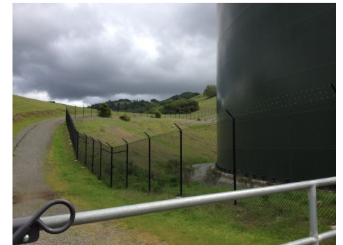
Kawana water tank, Taylor Mountain
