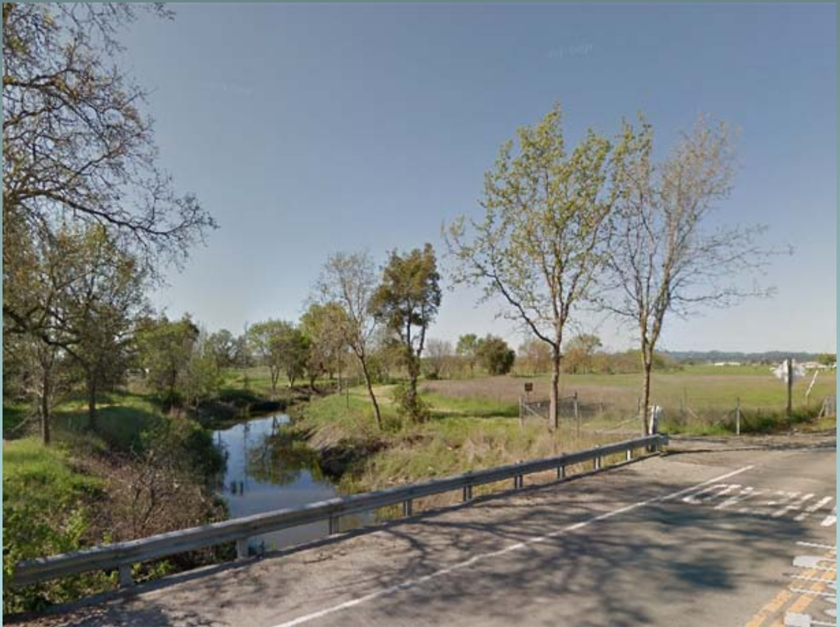
Colgan Creek, as it passes under Todd Road. The landscape is more open here, and is used partly for agriculture.
