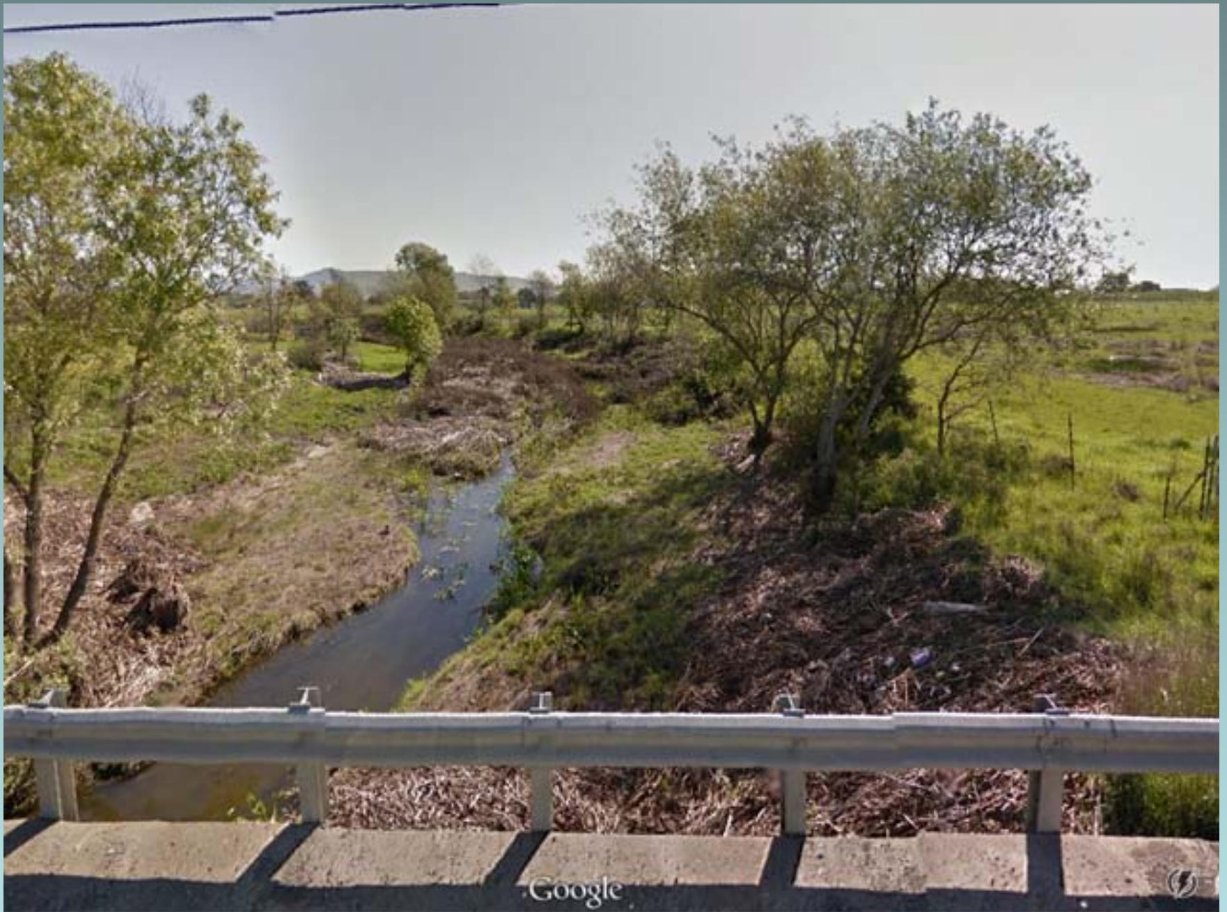
At Llano Road, looking upstream.
